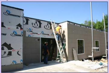
**STEP 5:** Special fiber-cement siding ( with 30 year warranty) is being installed to give the building exterior an architectural sandstone block appearance. The siding material can be applied directly on top of the concrete slab.
