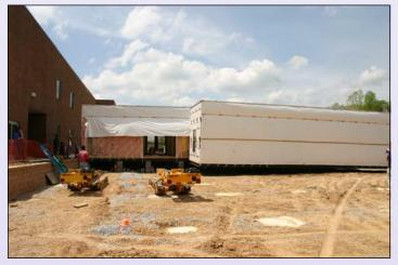
**STEP 2**: When the completed modules arrive on site from the factory, they are parked over the footings, then precisely maneuvered into place against the retaining wall by the setup crew using a Translift.
