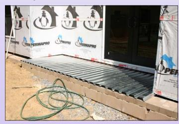
**STEP 4:** A piece of corrugated steel is placed from the recessed entry to the retaining wall. A poured concrete slab is then added to the entire entry area right up to the doorway.
