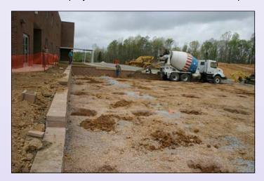
**STEP 1:** The site is prepared with a concrete retaining wall and poured concrete footings at the same time the building is being built at our climate controlled factory.
