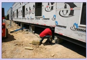
**STEP 3:** The setup process repeats until all modules arrive at the site. All the modules are blocked, leveled and strapped together.
