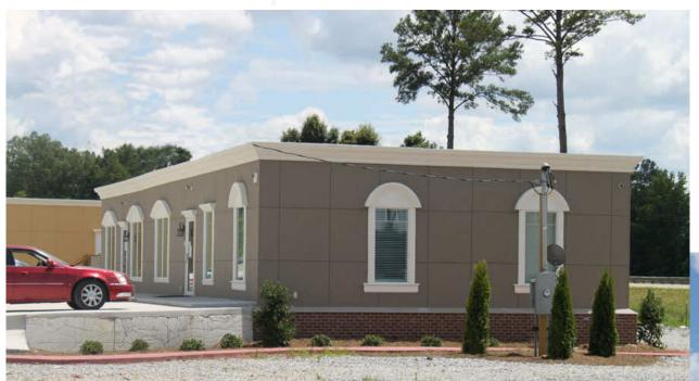
Finished building. Note that both of the exterior doors exit onto the side walk and parking lot with no ramps or steps. The middle picture shows the back side of building with the floor level approximately 36 inches off the ground.
