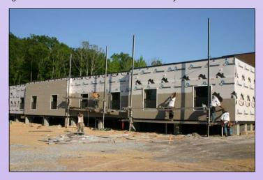
**STEP 5:** Special fiber-cement siding ( with 30 year warranty) is being installed to give the building exterior an architectural sandstone block appearance. This siding comes in a variety of finishes for a masonry look without the high cost. At the same time, the interior is being finished, painted, and carpeted.
