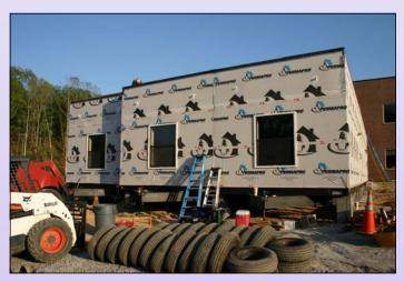
**STEP 3:** All modules are assembled, leveled, then securely anchored and bolted together to resist wind loads from 130 mph to over 150 mph in hurricane coastal zones. Transport gear is removed to be returned to the factory.
