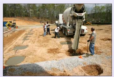
**STEP 1:** Poured concrete footings are being installed by Rose at the same time the building is being built at our large climate controlled factory. The site is prepared to receive the modules.
