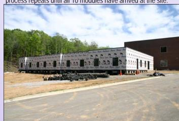
**STEP 4:** After all 10 modules have been assembled (this took 5 days) the building functions as one large 9,400 sq ft building instead of 10 individual modules. The interior and exterior finish work begins. Utilities are connected at this stage.
