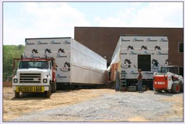
**STEP 2:** When the completed modules arrive on site from the factory, they are parked over the footings, then precisely maneuvered into place by the setup crew using a Translift. This process repeats until all 10 modules have arrived at the site.
