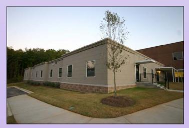
**STEP 6:** Once the siding and base is covered with the fibercement siding, a coping band is installed around the roof line to finish the exterior. This building has all the curb appeal and quality that you would find in a contractor built building, yet at a fraction of the cost. Normal completion time averages 90 to 120 days from starting. Also, it is expandable for future growth.
